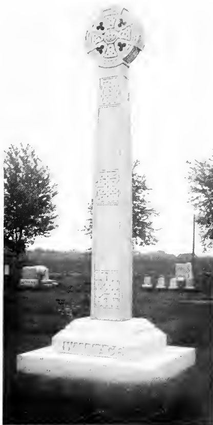
Number 8308. Still another English type as seen in Cornwall. Note how the slight expansion of the lines of the shaft at its centre, and its contraction as it approaches the nimbus, adds to its effectiveness. Special tooling gives it a pleasing, soft-textured effect. Erected at Ogdensburg, N. Y., for Mrs. Lew Wallace.
